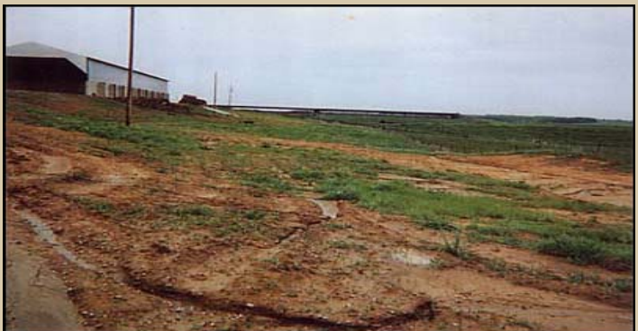
Lack of vegetative cover is accelerating erosion and runoff.
