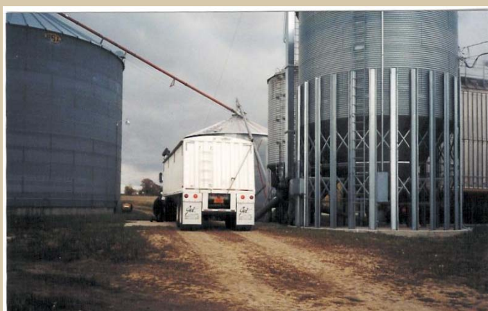
Debris free work area increases safety and efficiency.
