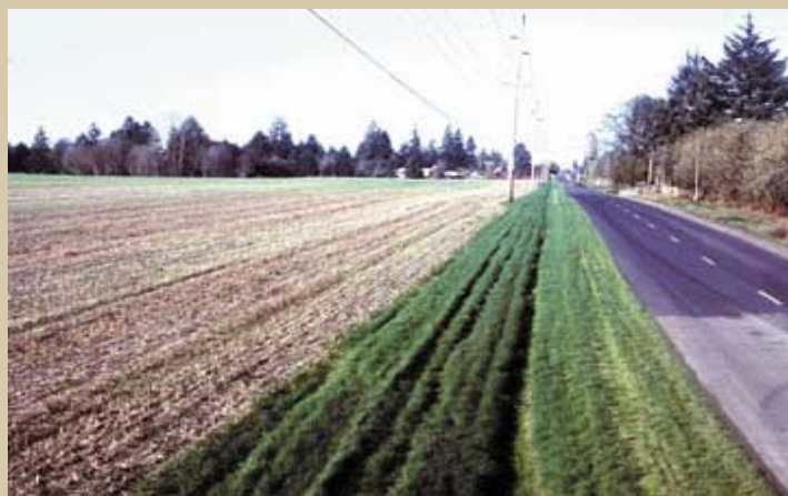
Well maintained ditch inhibits weeds and filters runoff.
