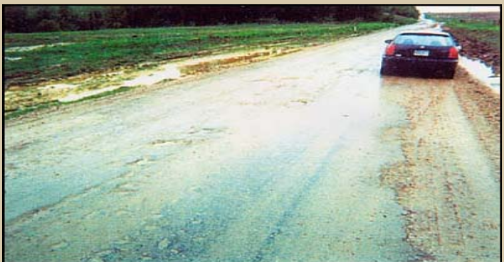
Spraying manure on the road is an obvious example of non-compliance.
