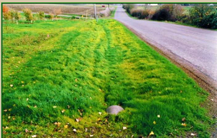
Wide, shallow ditch allows mowing and filters water from roads and fields.
