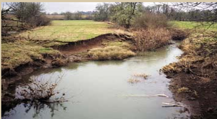
Banks that are not fenced off from grazing are prone to erosion.
